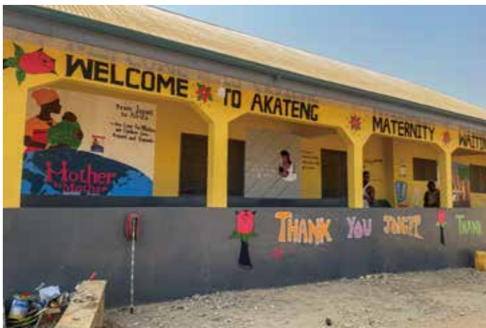
6. Completion of painting
